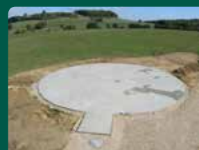
On-site base plate
