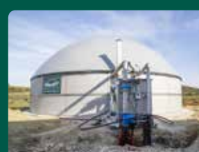
7. Day Pipeline construction completed and ready for operation
